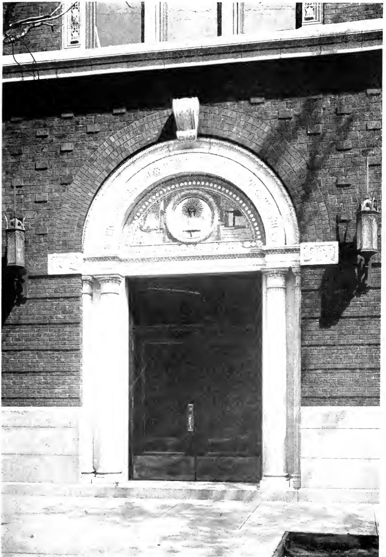
ENTRANCE DETAIL. BUILDING FOR THE AMERICAN BOOK CO., CHICAGO N. MAX DUNNING, ARCHITECT
